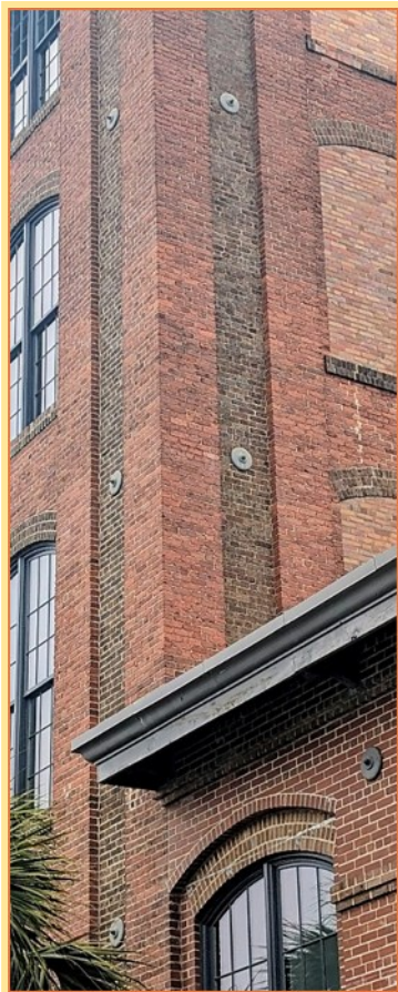
Above - Close-ups of the Old Cigar Factory's brickwork & earthquake bolts (rods). Photos by A.M. Shinault-Small
